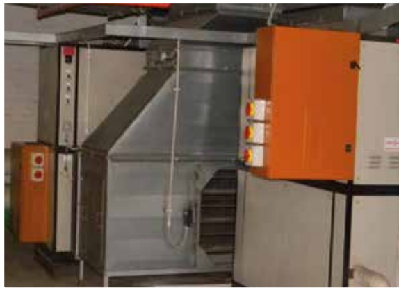
Air Handling Unit Plant and Air-Supply Fan
