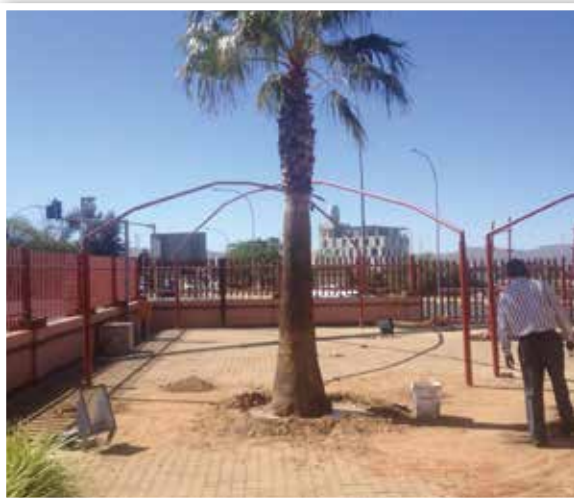
Construction of Shade-net Poles
