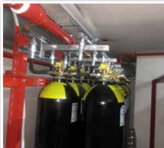
The gas fire suppression system (Pyroshield gas bottles)
