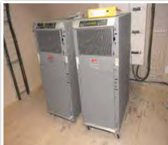
Newly installed UPS (un-interrupted power supply) units for IT
