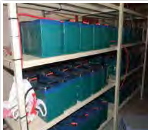
Newly installed battery bank for the UPS units
