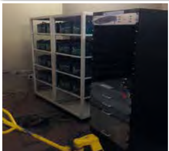
Installation of battery bank in progress
