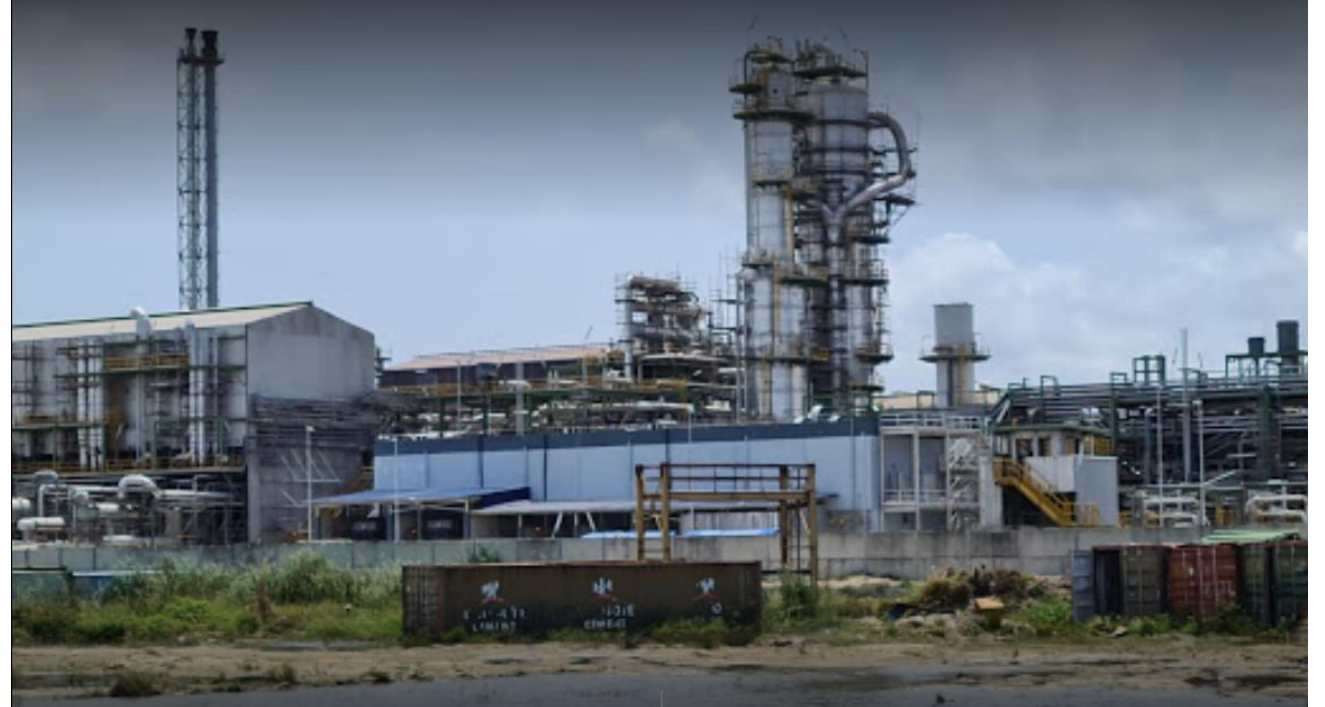
Dangote fertilizer plant (Nigeria). World's second largest urea plant with annual production 3 mill t/yr.
