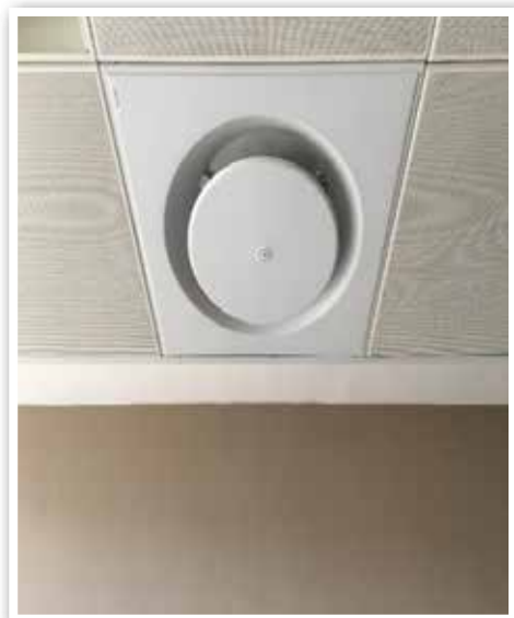
New energy-efficient diffusers installed on Floor 1
